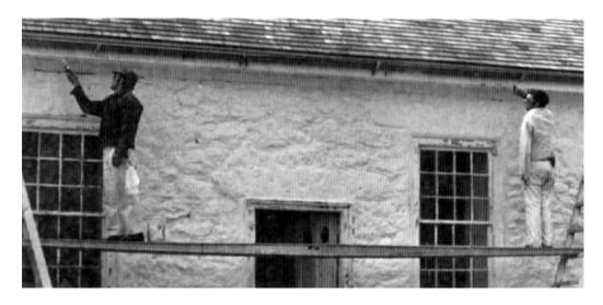
Adequate protection and maintenance of a historic building is an ongoing commitment. Here, two workers are priming and repainting exterior stone and wood trim. If surface treatments are neglected, more extensive repair and replacement will be required. Each loss further undermines a building's historic integrity.
