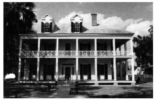
The Bronson-Mulholland House in Palatka, Florida, ca. 1845, is shown (a) before and (b) after the treatment, Restoration. Over the years the east (far right) side of the veranda had been filled in as a sixth bay. During the restoration, this later infill was removed and the east veranda, together with its flooring, stairs, and foundation, restored. Photo: City of Palatka, Community Development Department.
